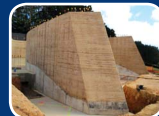
Foundations for the new Welcome Centre currently under construction.
